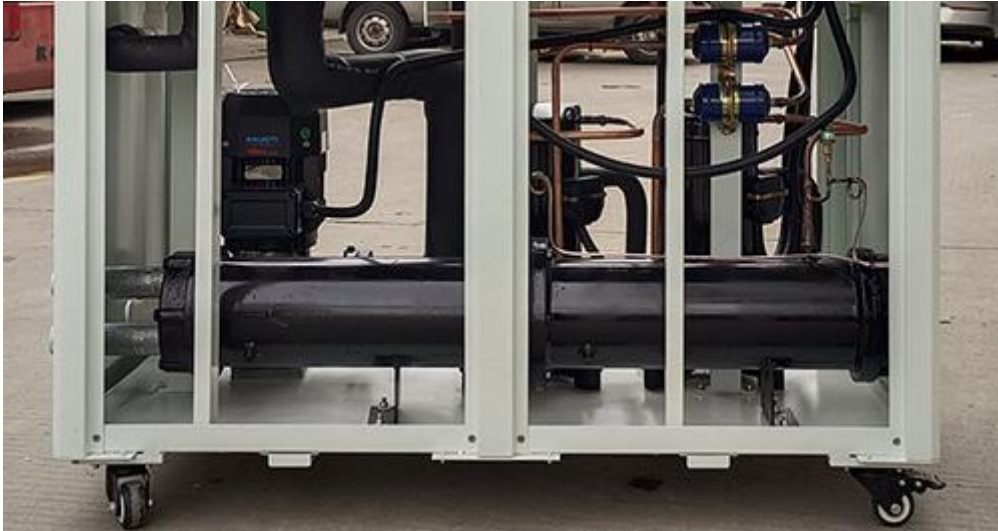
Shell and tube Condenser for water-cooled Plastic Processchiller
